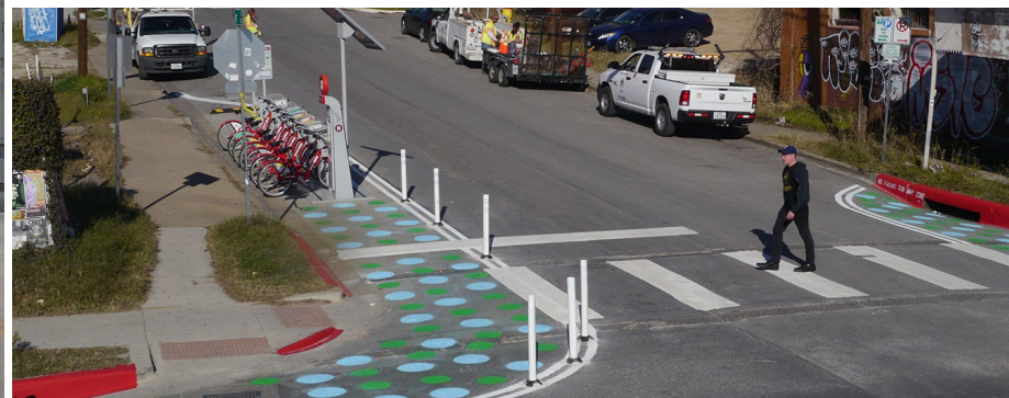
CURB EXTENSION CARVED OUT BY TEMPORARY MEASURES
