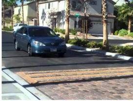
ROUNDABOUTS & RUMBLE STRIPS ALONG WITH PAVING DIFFERENCE AS TRAFFIC CALMING MEASURE
