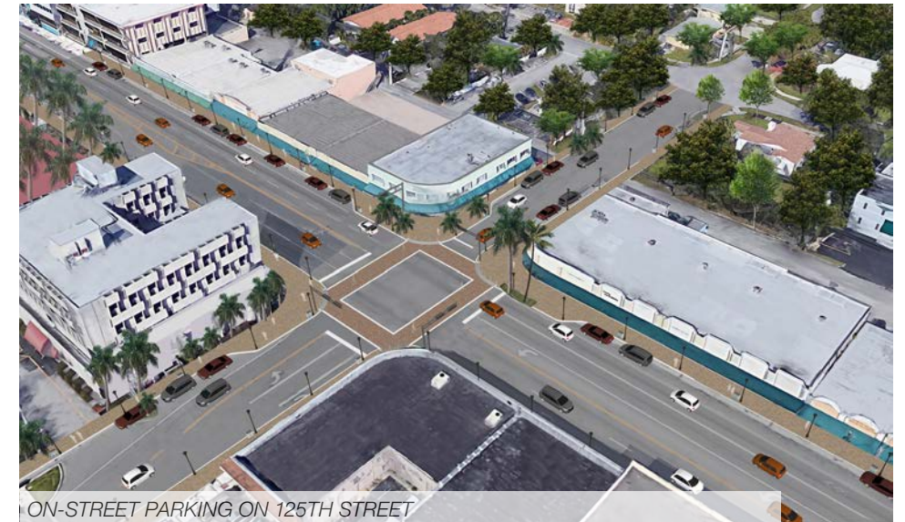
ON-STREET PARKING ON 125TH STREET
