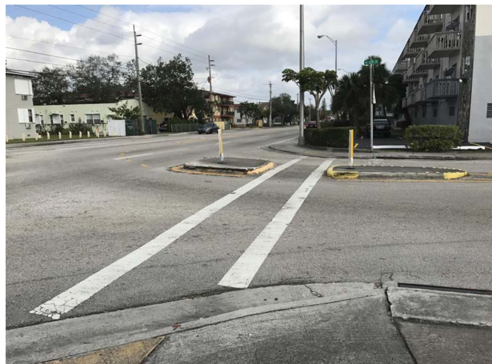
04 View towards North of NE 129th St. and East of NE 10th Ave.
