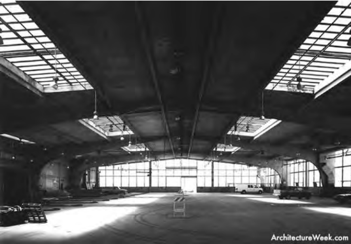
FORMER GREYHOUND BUS MAINTENANCE FACILITY
